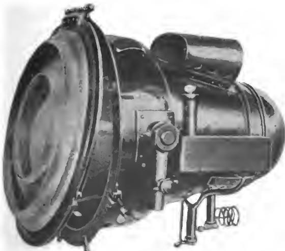
FIG. 5.—BLERIOT SEARCHLIGHT, BURNING GASOLINE AND OXYGEN. FIG. 6.—GRAND PROJECTOR, SHOWING ARRANGEMENT OF BURNER.
